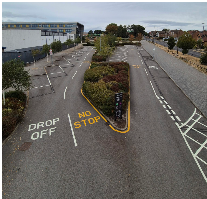
Figure 1: The Drop Off and No Stop lanes
